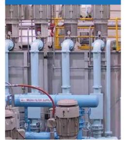
The two central coolant filter systems pictured were provided to Navistar International for the 6.0 liter V8 Diesel Engine Program.
